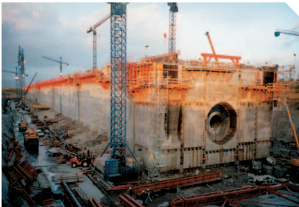
During construction in the dry shipyard in Southern Spain
