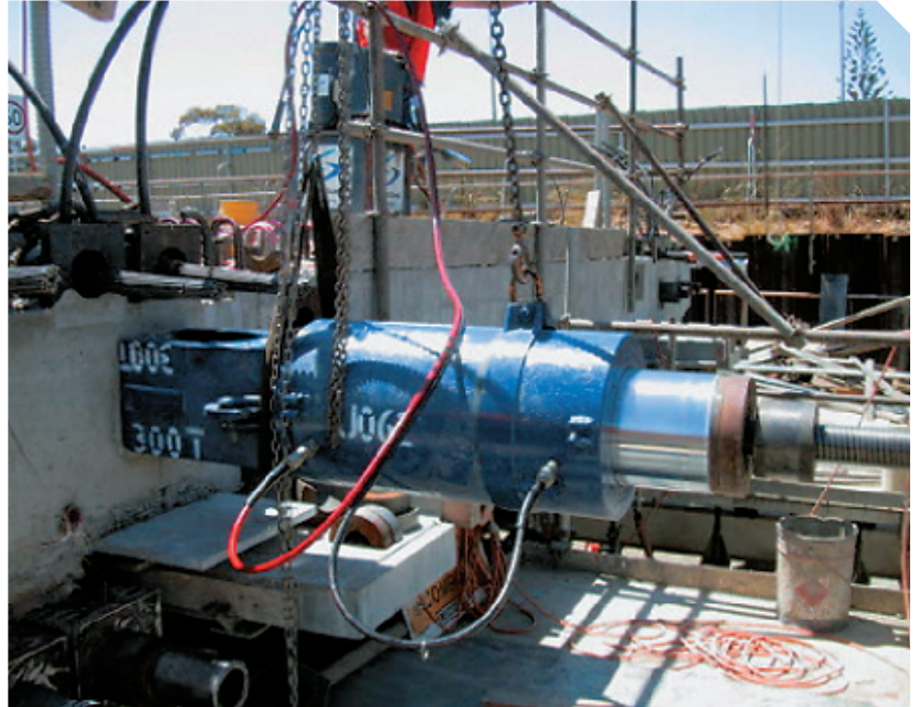
Stressing Jack in operation
