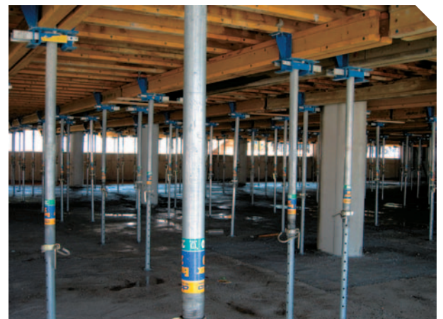
Formworks and propping
