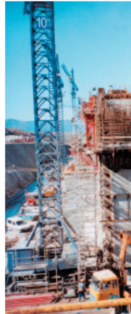
During construction in the dry shipyard
