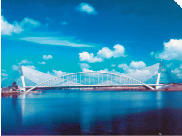
Bridge after the installation of Hangers and Stays
