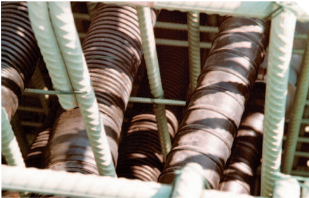
Plastic ducts in a congested rebar environment
