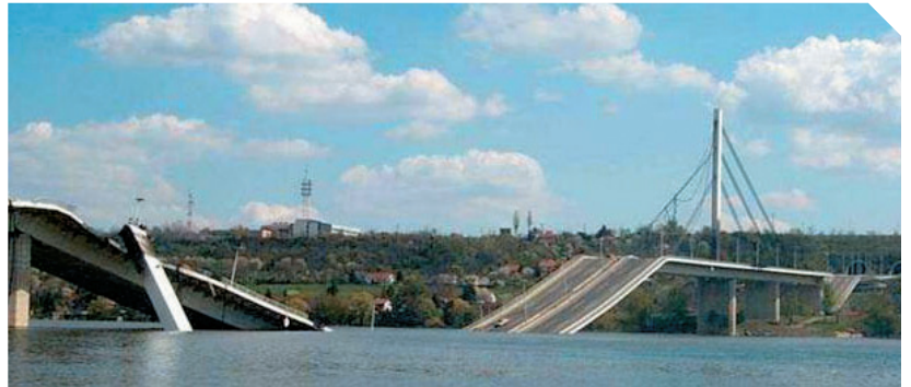
Collapsed Bridge after NATO attacks in April 1999
