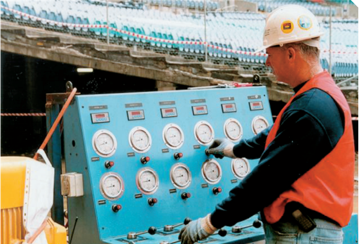
BBR fully automated control panel
