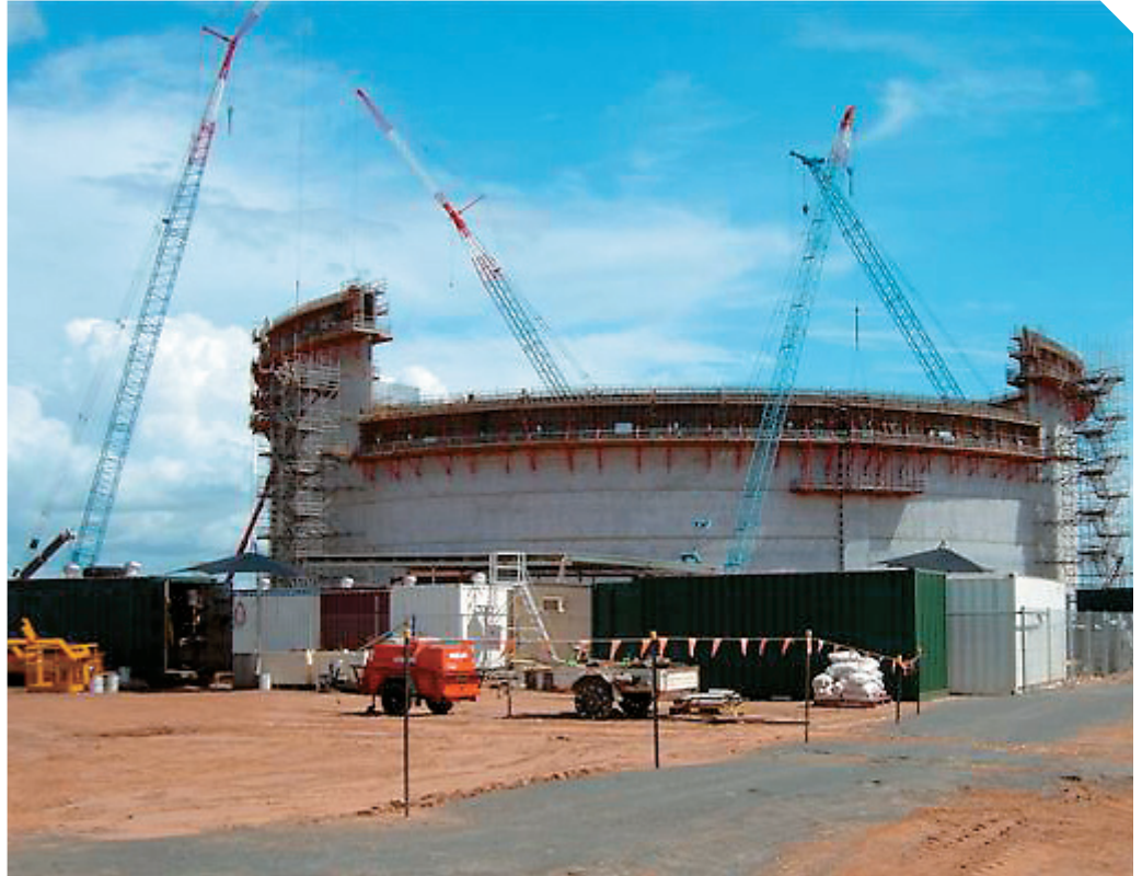
Tank under construction
