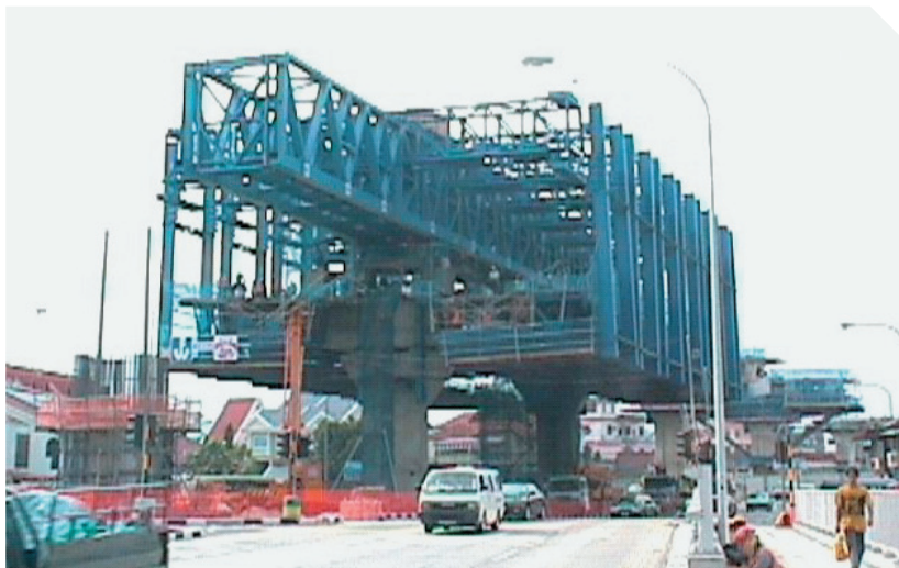
Advanced Launching Girder method
