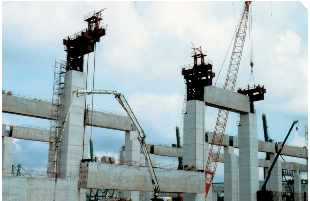
Heavy Lifting set up
