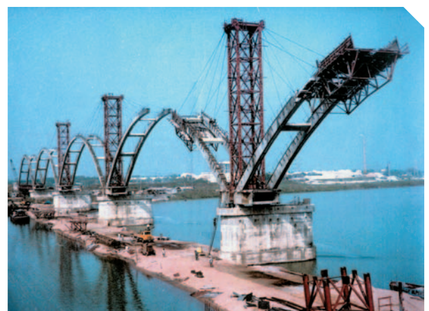
Godavari Bridge during construction
