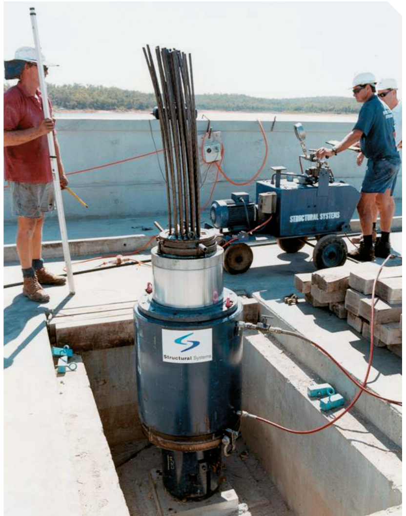
Stressing Jack under operation
