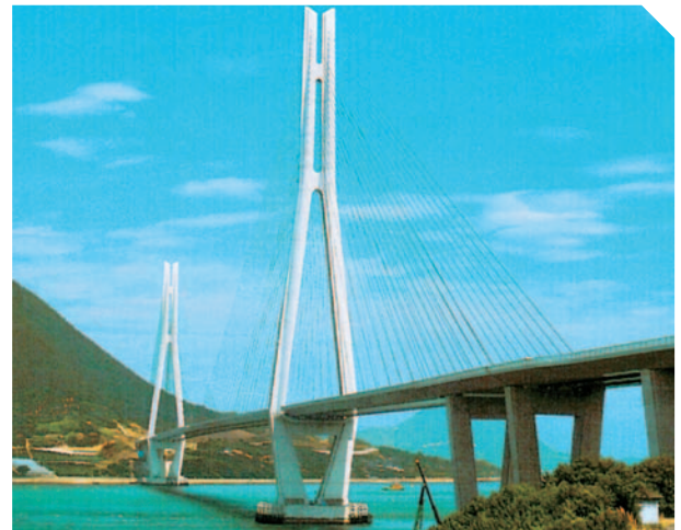
Tataro Bridge, Japan
