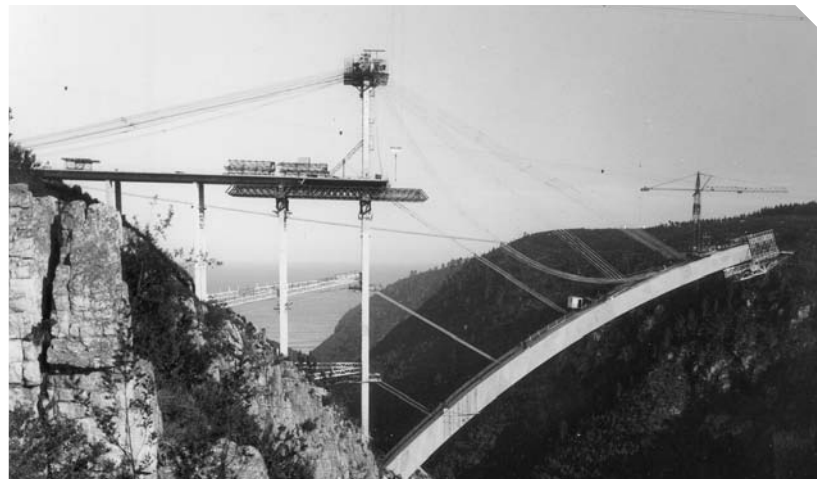
Temporary works, Bloukrans Bridge
