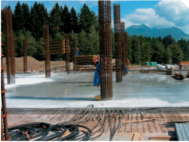
Curing of the concreted plot
