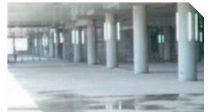
View inside the Main Building (Head House 01B)
