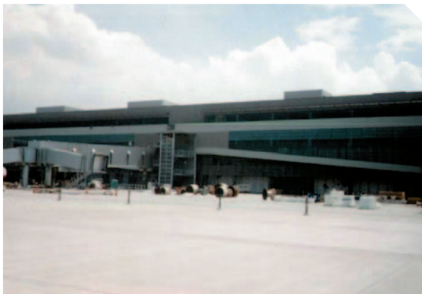
The completed Main Buildings
