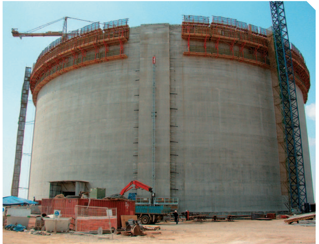
Tank during construction
