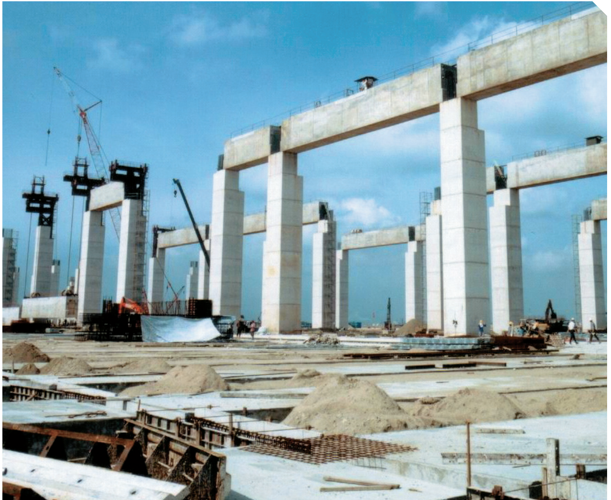
Erection of the beams
