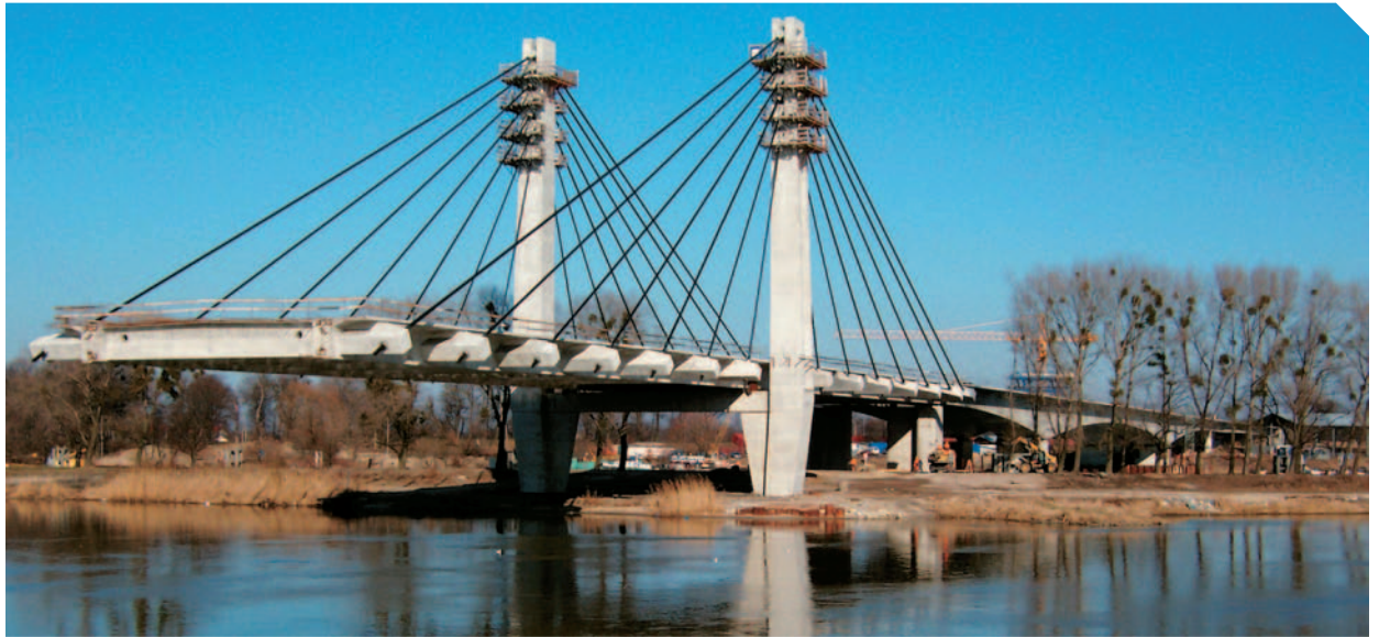
Millenium Bridge – view of the stay cable portion under construction
