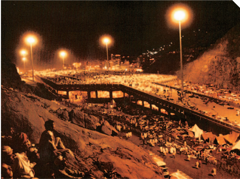
Mecca. Al Jamarat pedestrian bridge built on 3600 pieces of Proceq LASTO Block bearings
