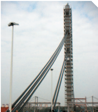
Installation of new BBR CONA STAY Cables
