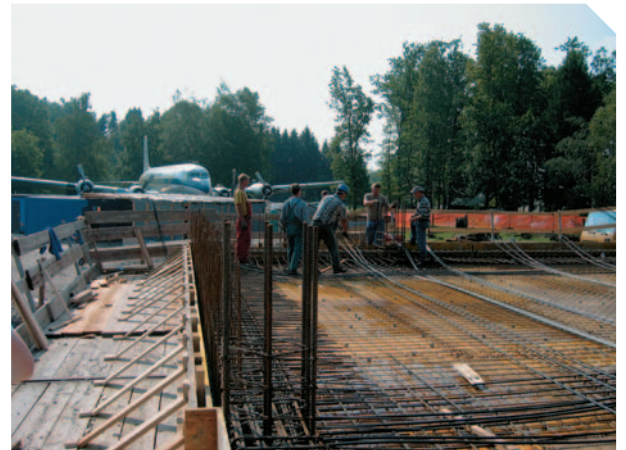
PT layout at stressing end
