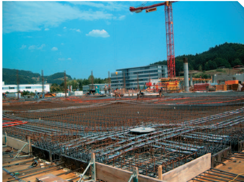
General view of the PT flat slab
