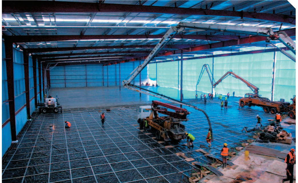
Casting of the slab
