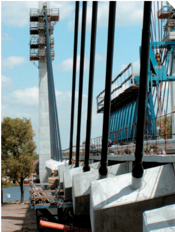
Detail of the deck anchorage zone
