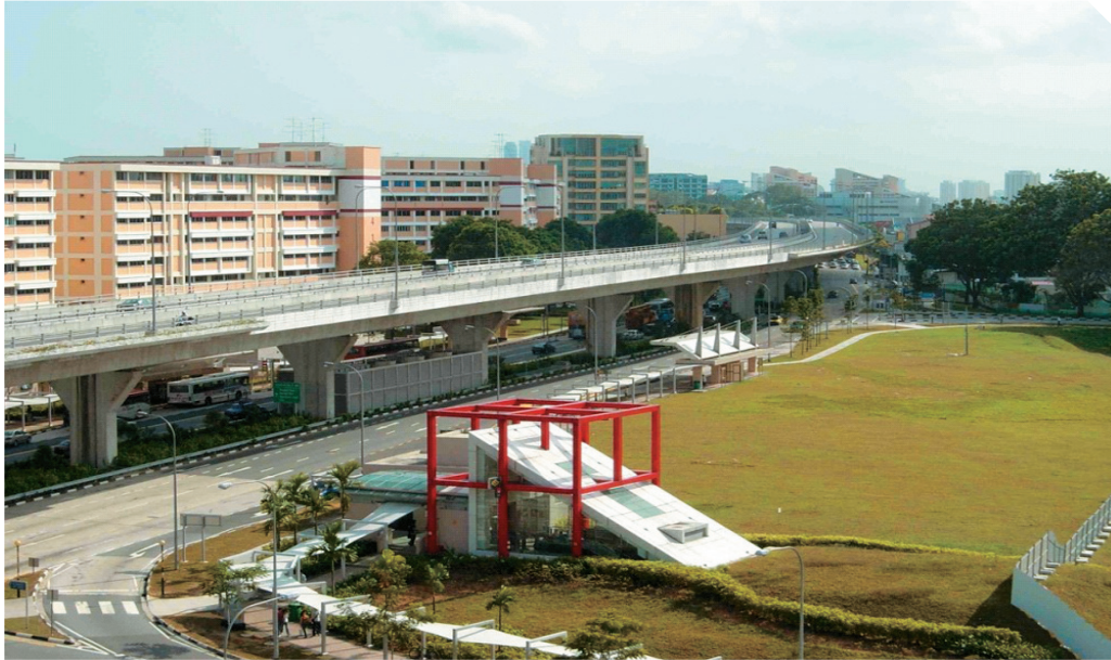
View of Middle Stretch of the Viaduct
