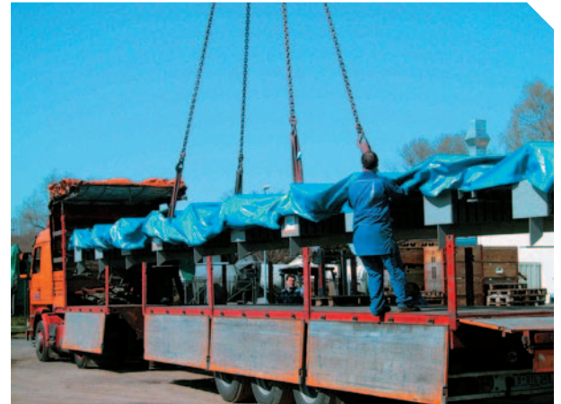
Unloading of the expansion joint
