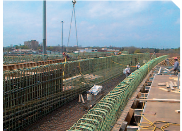
Reinforcement of the Segmental Bridge
