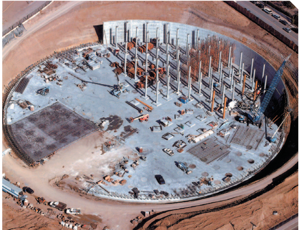
Roof slab pouring sequence
