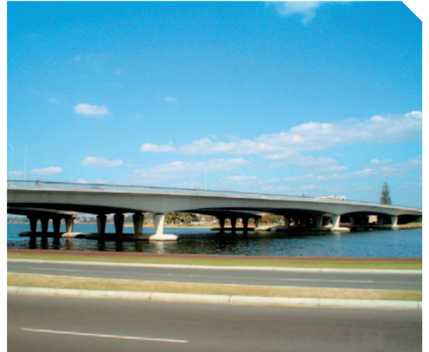
Bridge after finishing works
