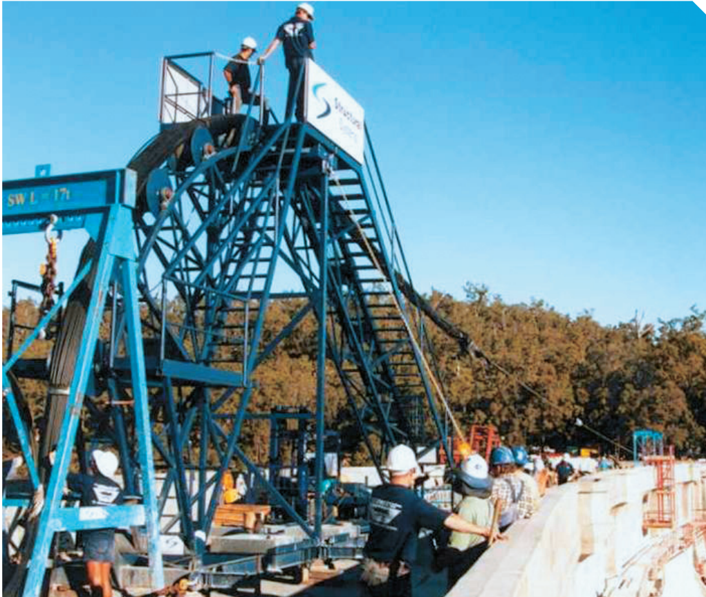
BBR Cona Sol installation
