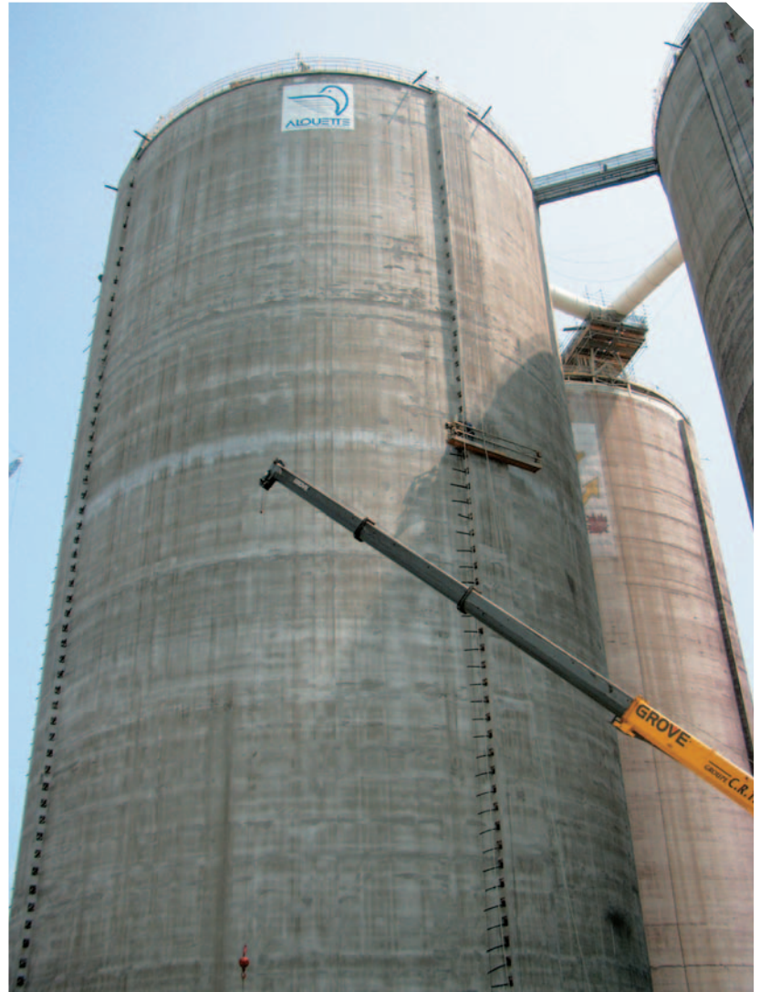
View of the four Alouette Silos
