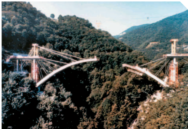
Arch of Val Crotta-Bridge during construction
