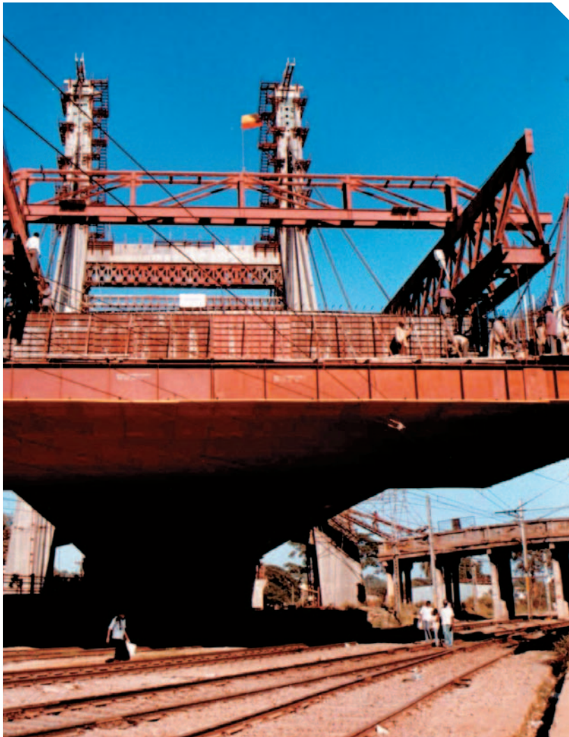
Cantilever Form Traveller suspended from BBR Dina Cables
