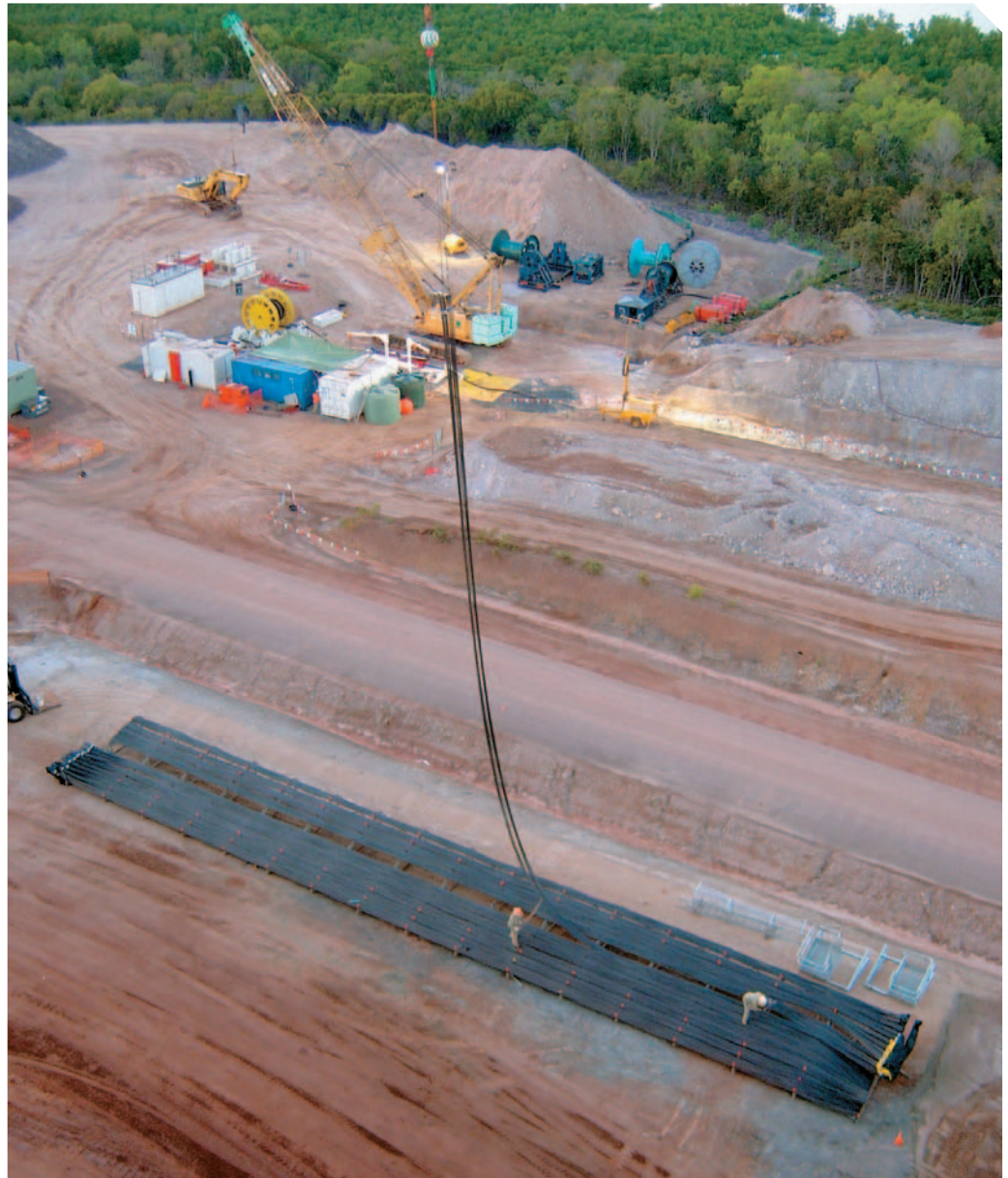
Strand lifting operation
