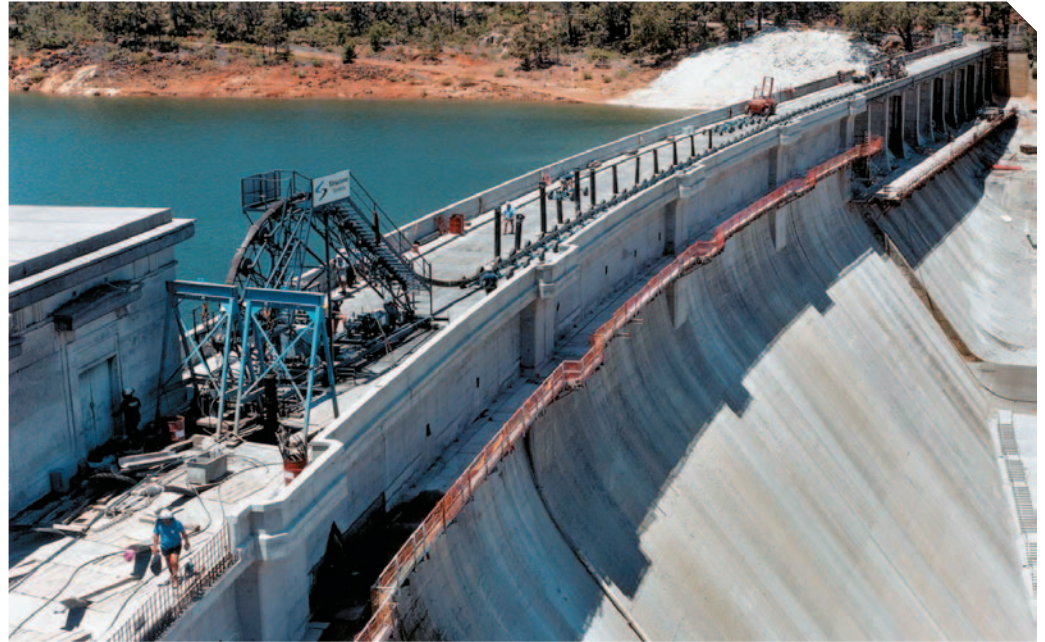
View of the installation setup
