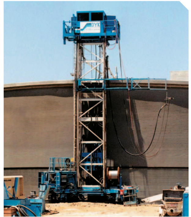
BBR automated strand winding machine
