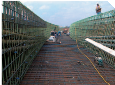
View into the Bridge Deck Section with PT ducts
