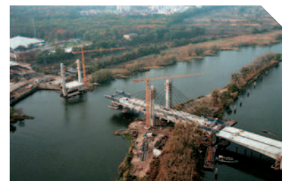
Formwork carrier shortly before closing pour
