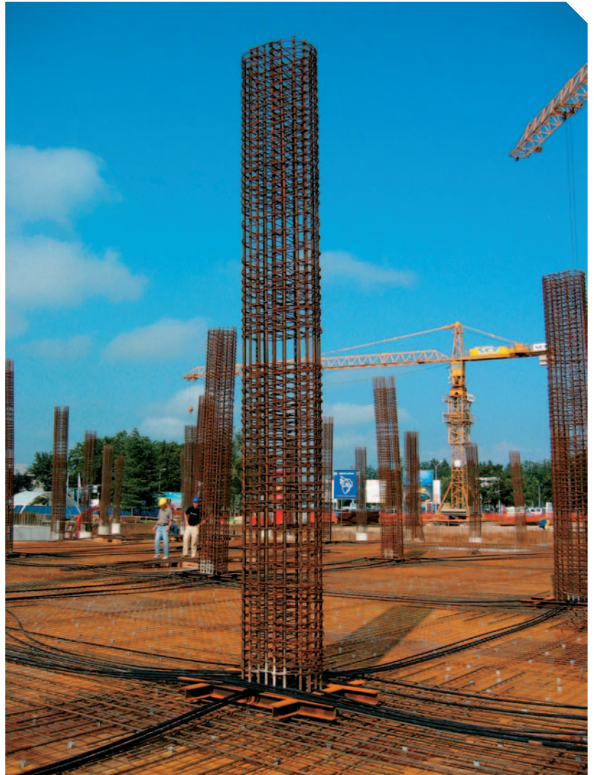
Detail of PT layout under the column
