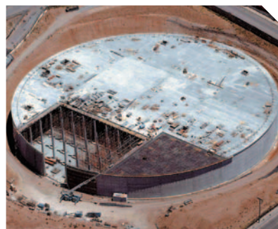
Erection of columns
