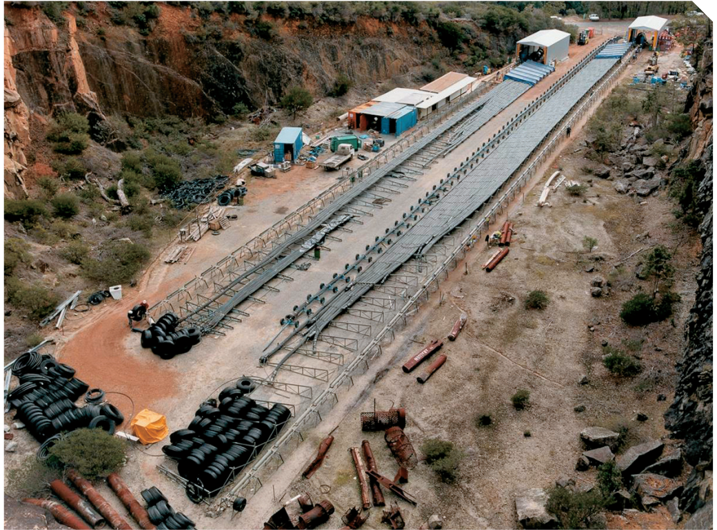
BBR Cona Sol preparation
